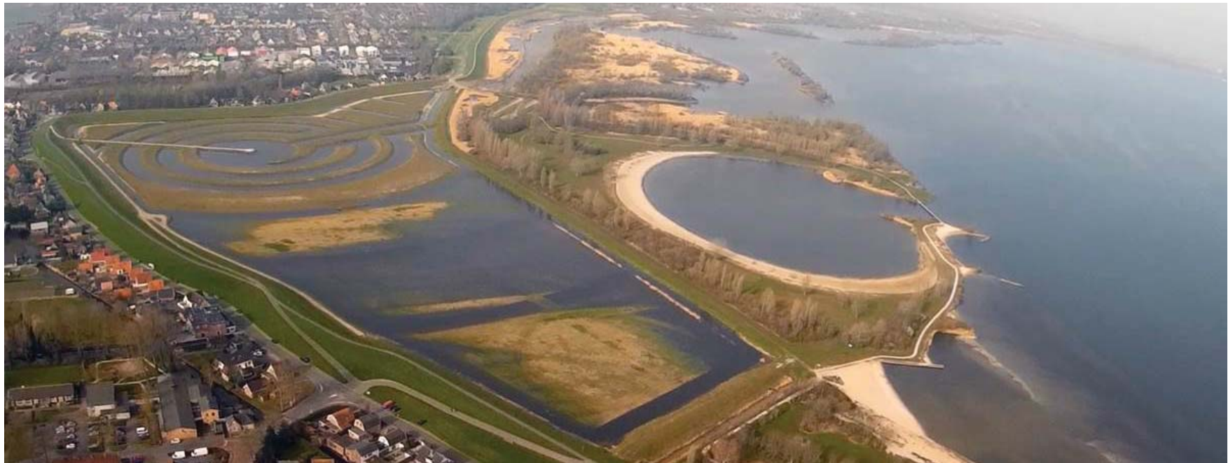
Recent construction of Markerwadden in the former Zuiderzee near Amsterdam: creating nature, supporting recreation and improving water quality, an example of a second berm concept.
